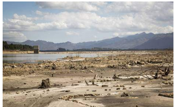
Theewaterskloof Dam near Cape Town, 6 May 2016.
